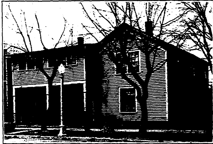
THE MAIN PORTION OF THIS BUILDING SERVED AS THE PUBLIC SCHOOL FROM 1865 TO THE EARLY 70's.
