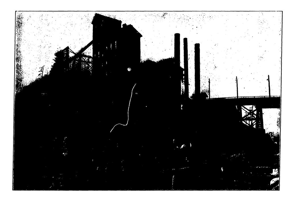
GENERAL view of Furnace Plant. From left to right the major objects shown are four stoves for heating the blast, the cast-house, the furnace proper, boiler chimneys, part of the stock-house, and ore roaster chimney.
