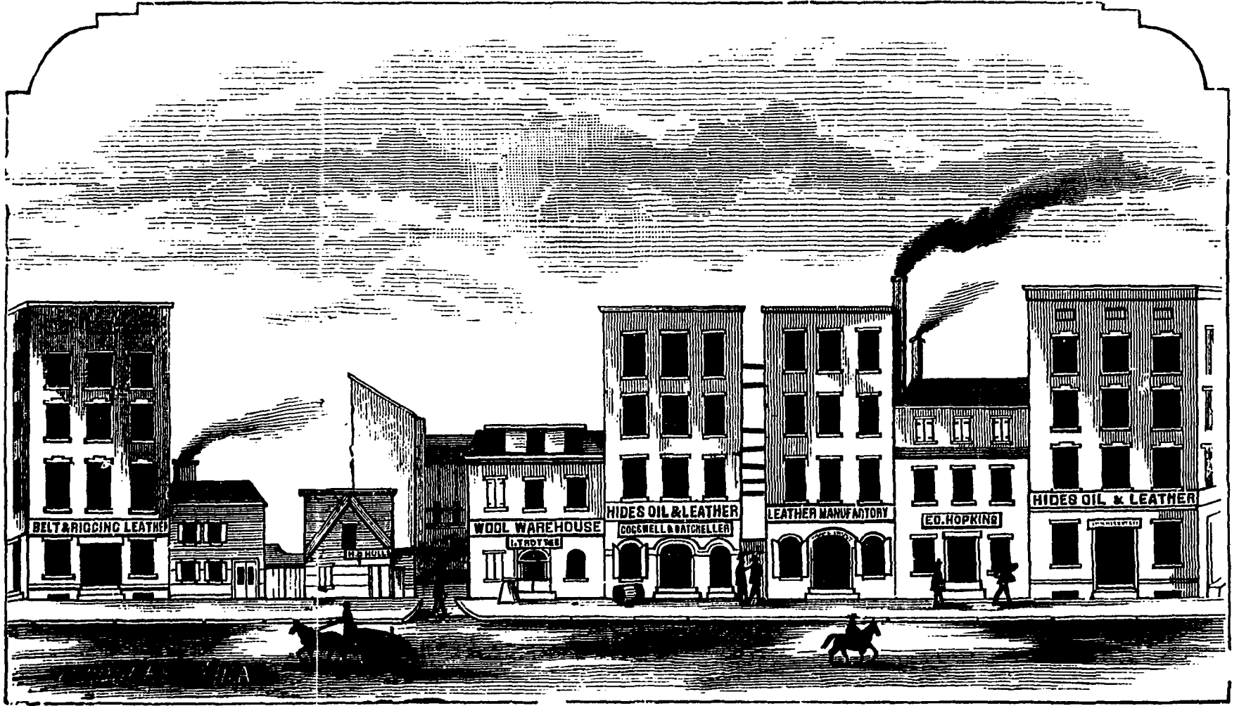
VIEW OF FERRY STREET, NORTH SIDE, 1840. LOOKING DOWN TO CLIFF STREET.
