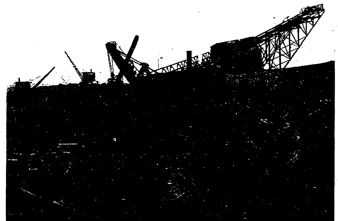
A PORTION OF THE DREDGING WORK NOW BEING DONE AT LOCKPORT FOR THE NEW 1,000-TON BARGE CANAL
