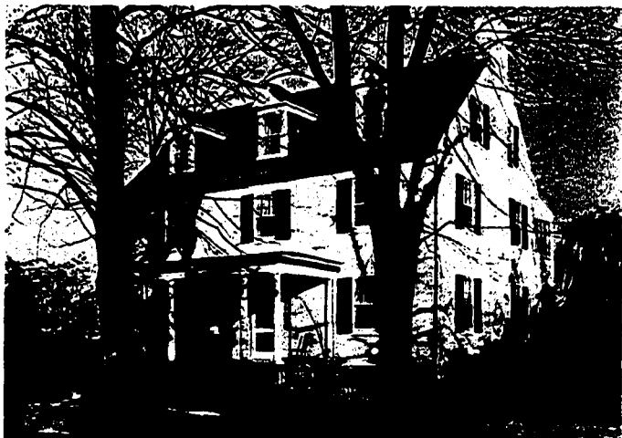
"320 NORTH KING STREET, LEESBURG, VIRGINIA Home of Mr. and Mrs. Ellsworth Marshall Rust, and built by them in 1918. View of front from southwest.
