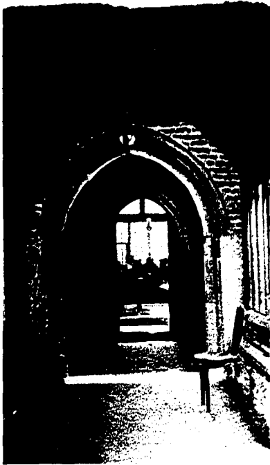
Main Entrance, Yaldam House
