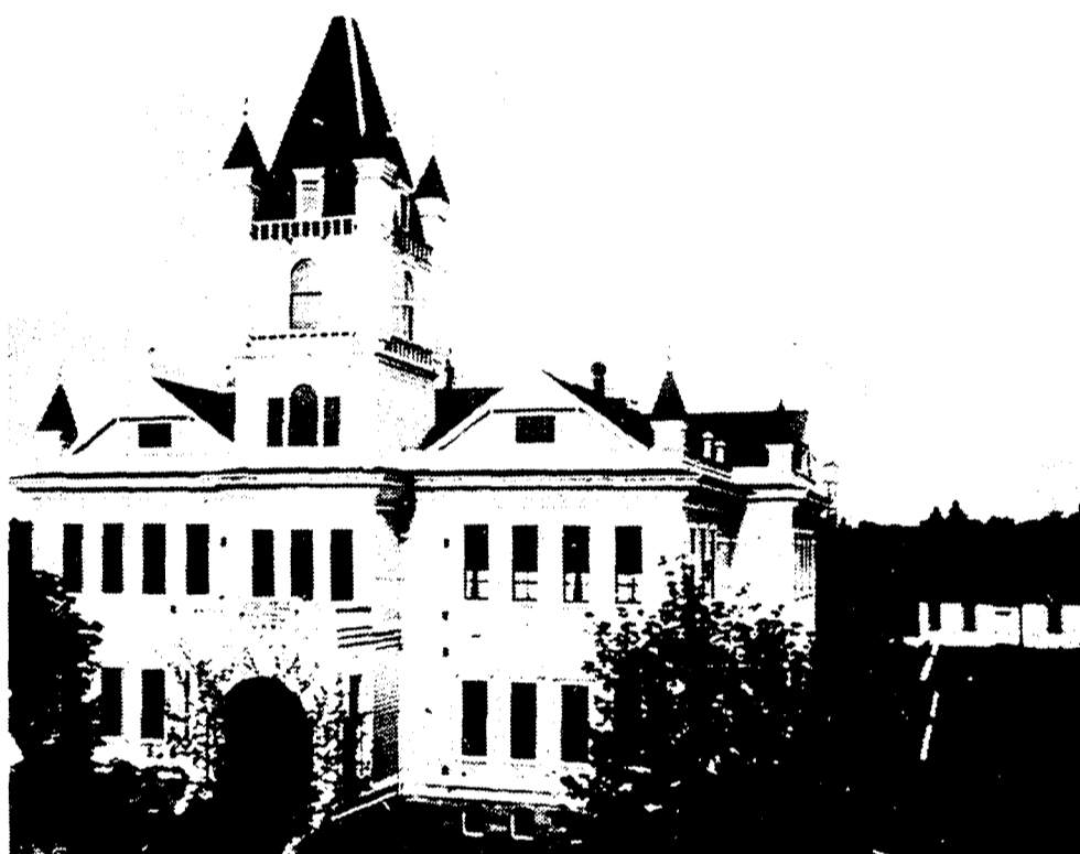
Clinton Kelly Elementary School erected in 1892 and razed in 1929, with No. 2 School in right background.
