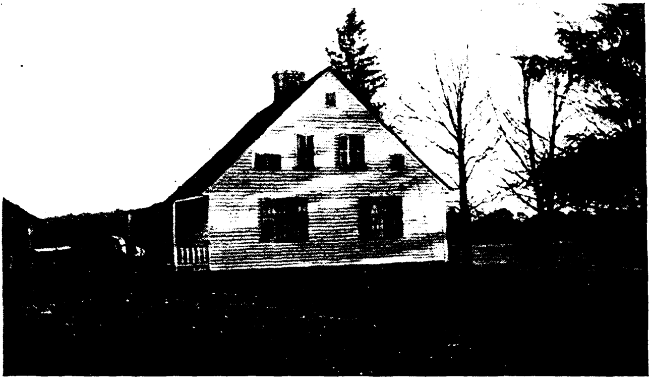
SELA WILCOX HOUSE, CLINTON
