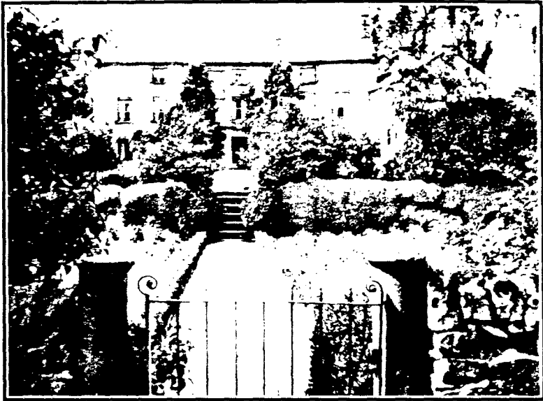
RESIDENCE OF MAJOR JOHN ELEY. IN 1790, AT ALPORT, DERBYSHIRE From photograph taken in 1903
