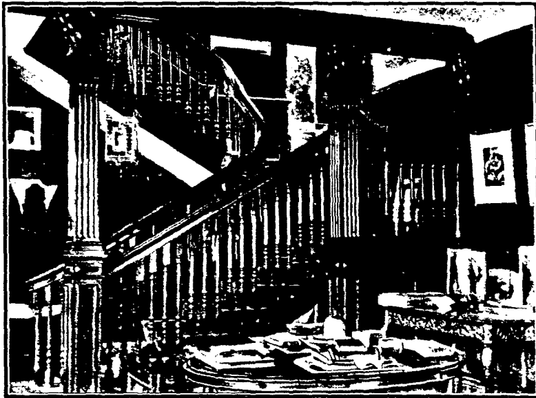
INTERIOR VIEW OF MANOR HOUSE, UTTERBY
