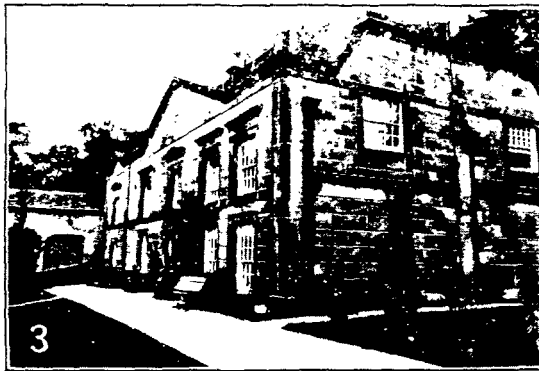
1. OGSTON HALL 2. ANCIENT CHAPEL AT OGSTON 3. REVELL GRANGE From photographs 1903
